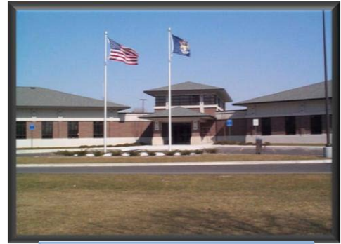
Georgetown Township Office
