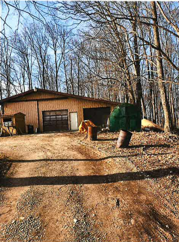
Front of pole barn looking north
